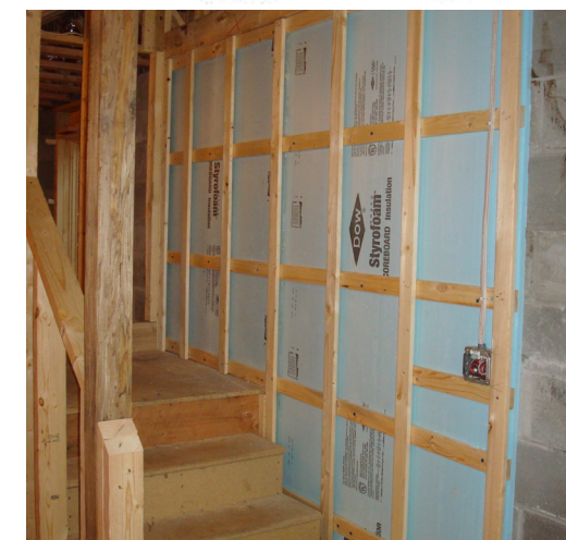
Basement framing system
