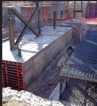
FOUNDATION BALLAST ©MCGOUGH
