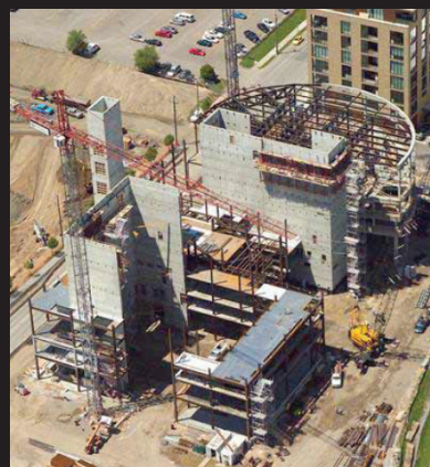
CONCRETE CORES AND STRUCTURAL STEEL ©MCGOUGH
