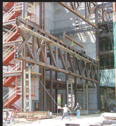
STEEL TRUSS TO SPAN OVER PROSCENIUM ROOF ©MCGOUGH
