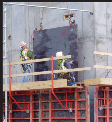
DOUBLE CONCRETE WALL CONSTRUCTION ©MCGOUGH
