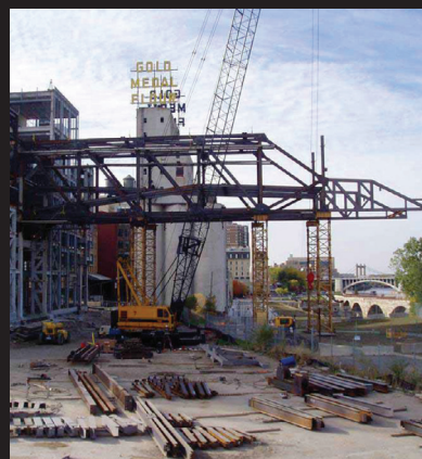
CANTILEVER CONSTRUCTION ©MCGOUGH
