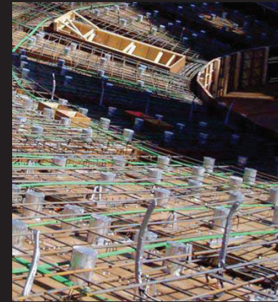
VENTILATION THROUGH THRUST SEATS ©MCGOUGH
